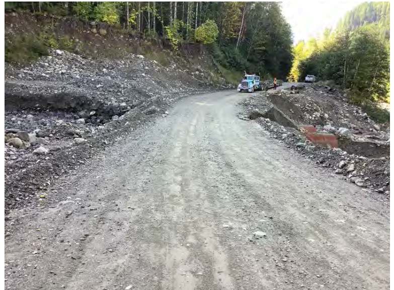
Approach from Right Bank when facing downstream
